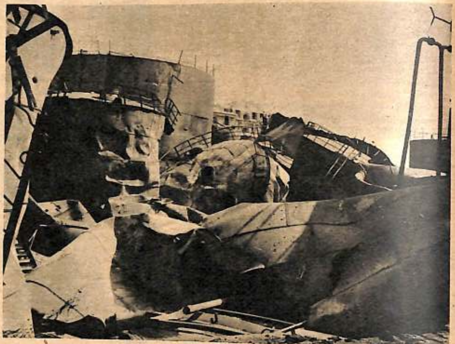
AMERICAN STRATEGIC BOMBING COST THE GERMANS 13,000 TONS OF OIL AND 29 VAST STORAGE TANKS AT GENNEVILLIERS. TANKS IN THE FOREGROUND BUCKLED FROM THE HEAT.
