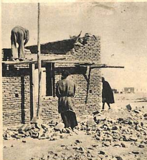
Natives work on an important building, the PX.
