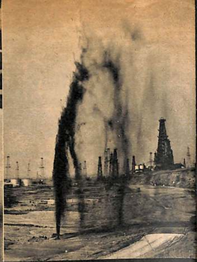
BEACH BATH. Oil fields at Huntington Beach, Calif., gushed steam, gas, mud and water erupting from sub-surface gas pockets.
