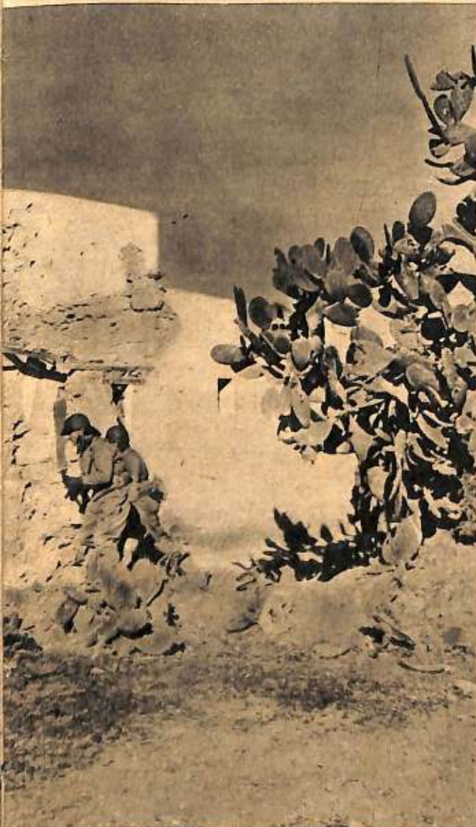
PAST A BATTERED BUILDING NEAR SENED.
