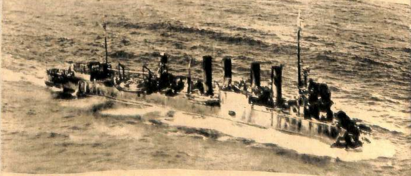
CASUALTY. The U.S.S. Blakeley, her bow blown off by an Axis torpedo, managed to plow into a Caribbean port for repairs, then made a 2,000-mile journey to Philadelphia, where a new bow was grafted on her. She's back on the high seas now, in good shape.
