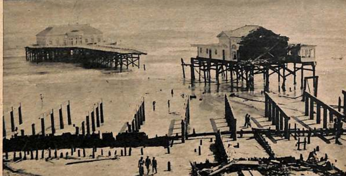
Here's how the Eastern Seaboard hurricane sliced Atlantic City's Heinz Pier, a landmark of the New Jersey resort. The Steel Pier, boardwalks and other amusement spots also suffered severe damage.
