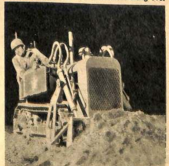
Creating an emergency airfield at night.
