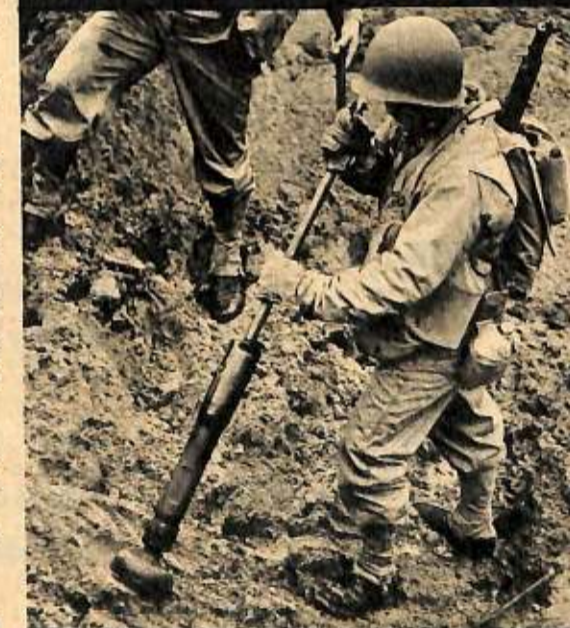
4. Pneumatic rammer packs down dirt in bomb hole.
