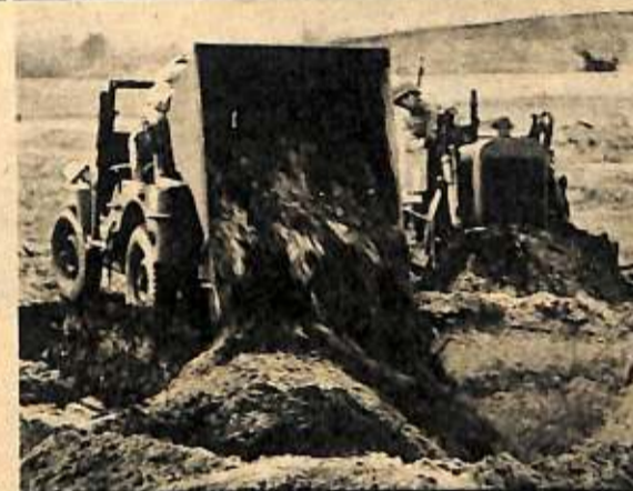
3. Quickly, jeep-dumper and scraper fill crater.
