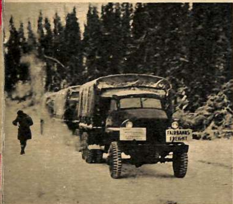
OPENING. Shortly after dedication of Alcan Highway, first army truck convoy carries war supplies to Fairbanks, Alaska.
