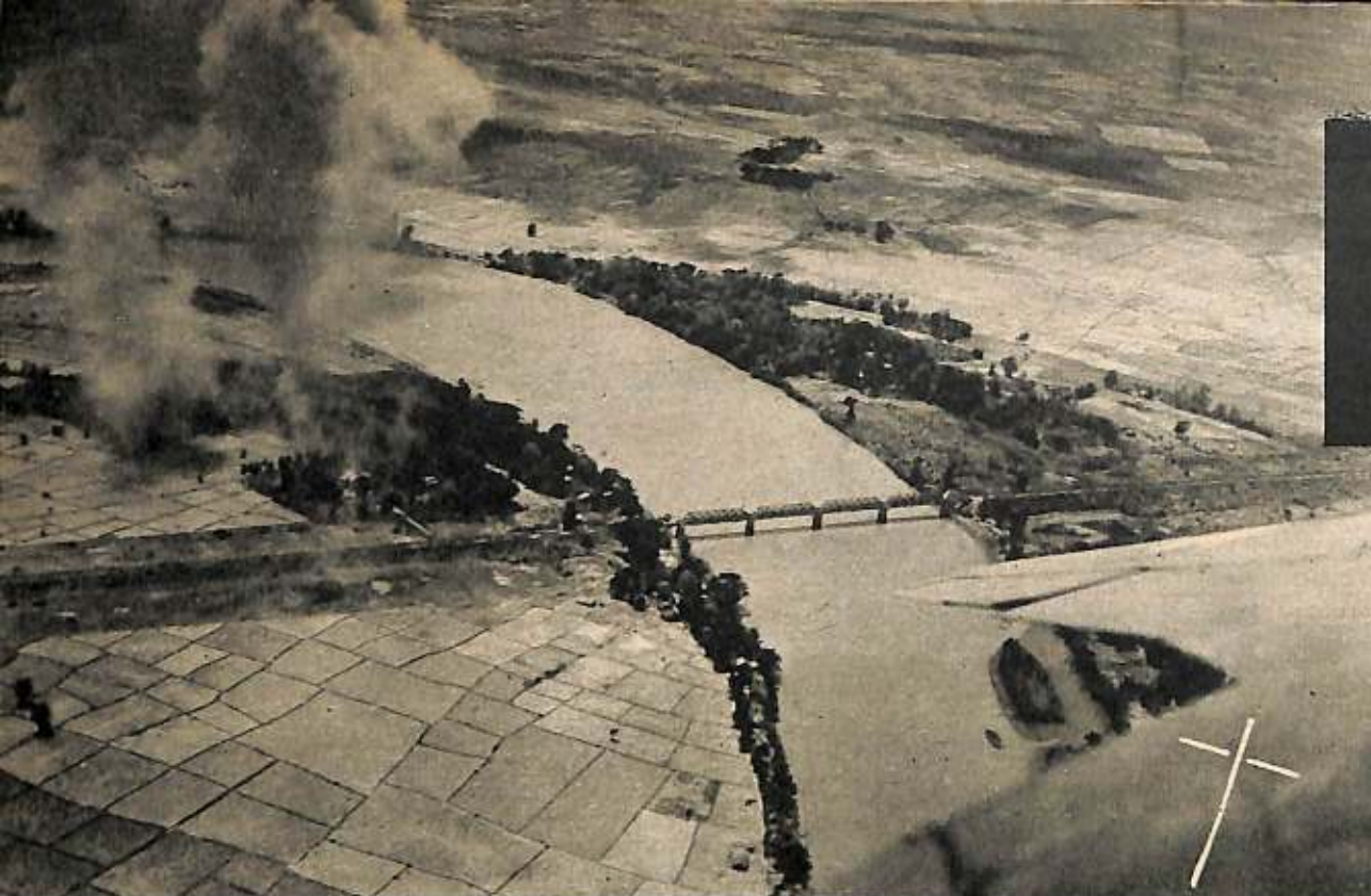
This is what the Daga River railroad bridge looked like before the Burma Bridge Busters went after it.
