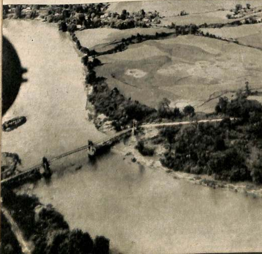
The Hsipaw bridge intact and an aid to the enemy before the B-25s attacked.
