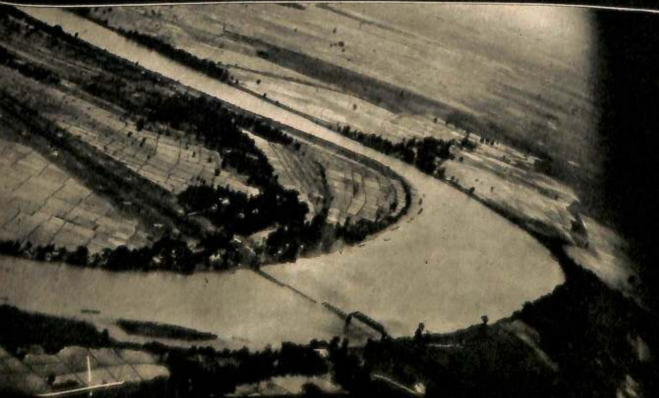
As the bombers flew back to their field they left the Daga bridge with three of its four trestles smashed.
