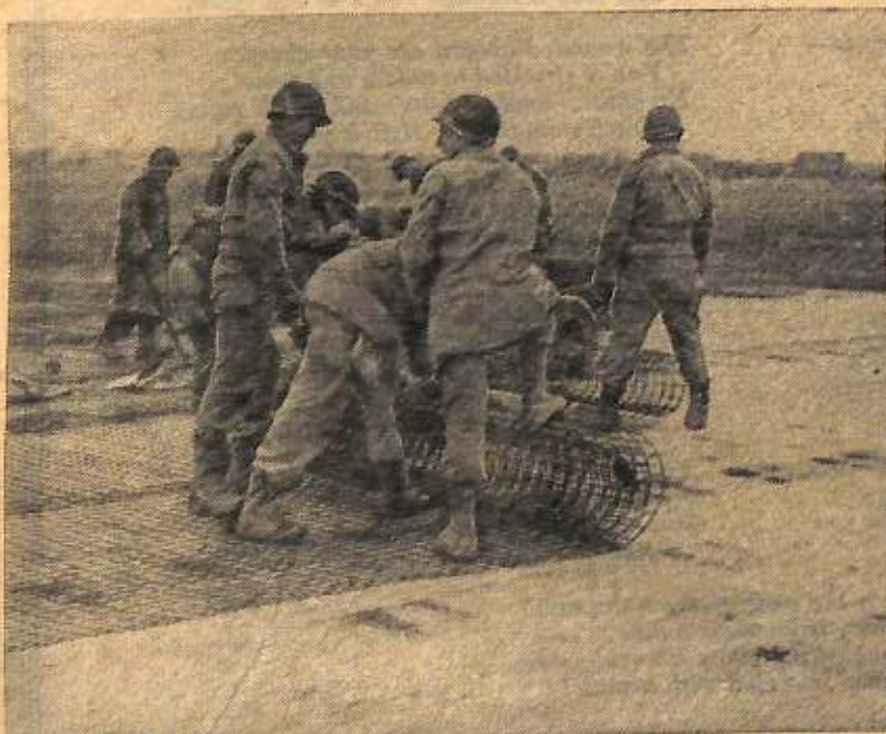
U.S. AVIATION Engineers unroll wire mesh over a landing field in Germany.
