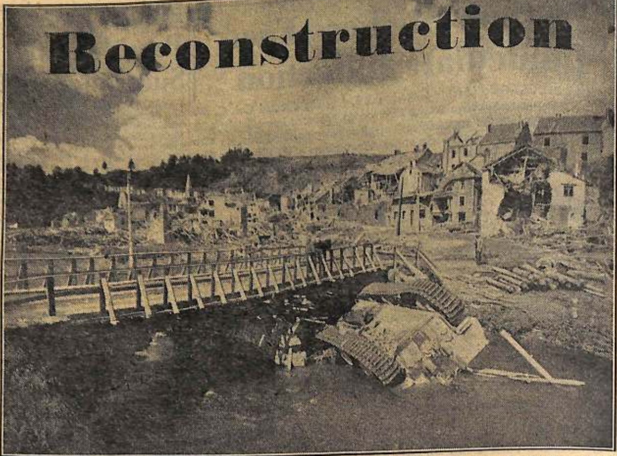
Out of the debris in the war-ravaged Ardennes, where von Rundstedt staged his ill-fated breakthrough last December, begins the hard job of reconstruction. Above is pictured an overturned German tank resting in a shallow stream alongside a rebuilt bridge in Houffalize, Belgium.
