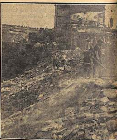
HOUFFALIZE: On one of the historical storage proceeds. Belg
