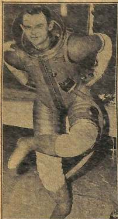
The Buck Rogers getup is the new flexible pressurized "strato-suit" of rubberized fabric developed at Akron, O., for high-altitude flying. Oxygen for breathing, sound for microphone and earphone connections and electricity for heated underwear are piped in through one assembly.
