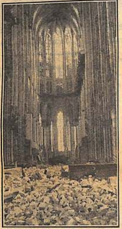
Large stone fragments, blasted loose during Allied air attacks on nearby targets, litter the floor of the Cologne Cathedral. Despite blast damage, the edifice remained structurally intact.
